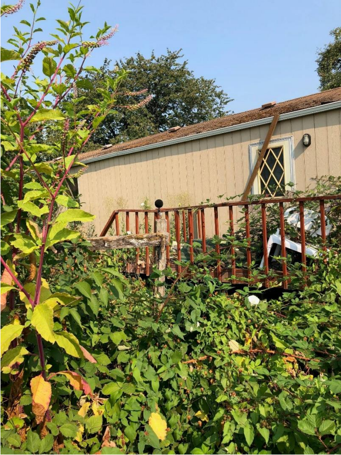
LT Site 1: 303 Hazel Street Picture 2 West
