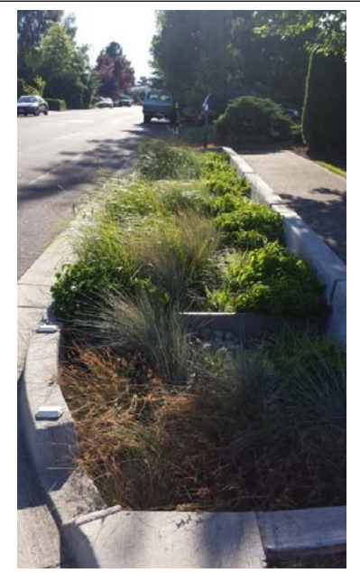
An example of a bioretention area built to capture street runoff. (Photo by Otak, Inc.)
