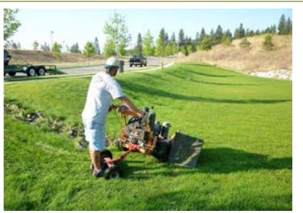
Illustrations of ongoing stormwater facility maintenance (photos are courtesy of Department of Ecology and AHBL, Inc.)
